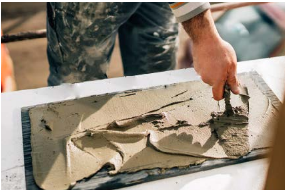
Fig. 3: generously back butter the stone.
